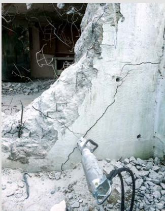
Demolition of concrete and reinforced concrete
